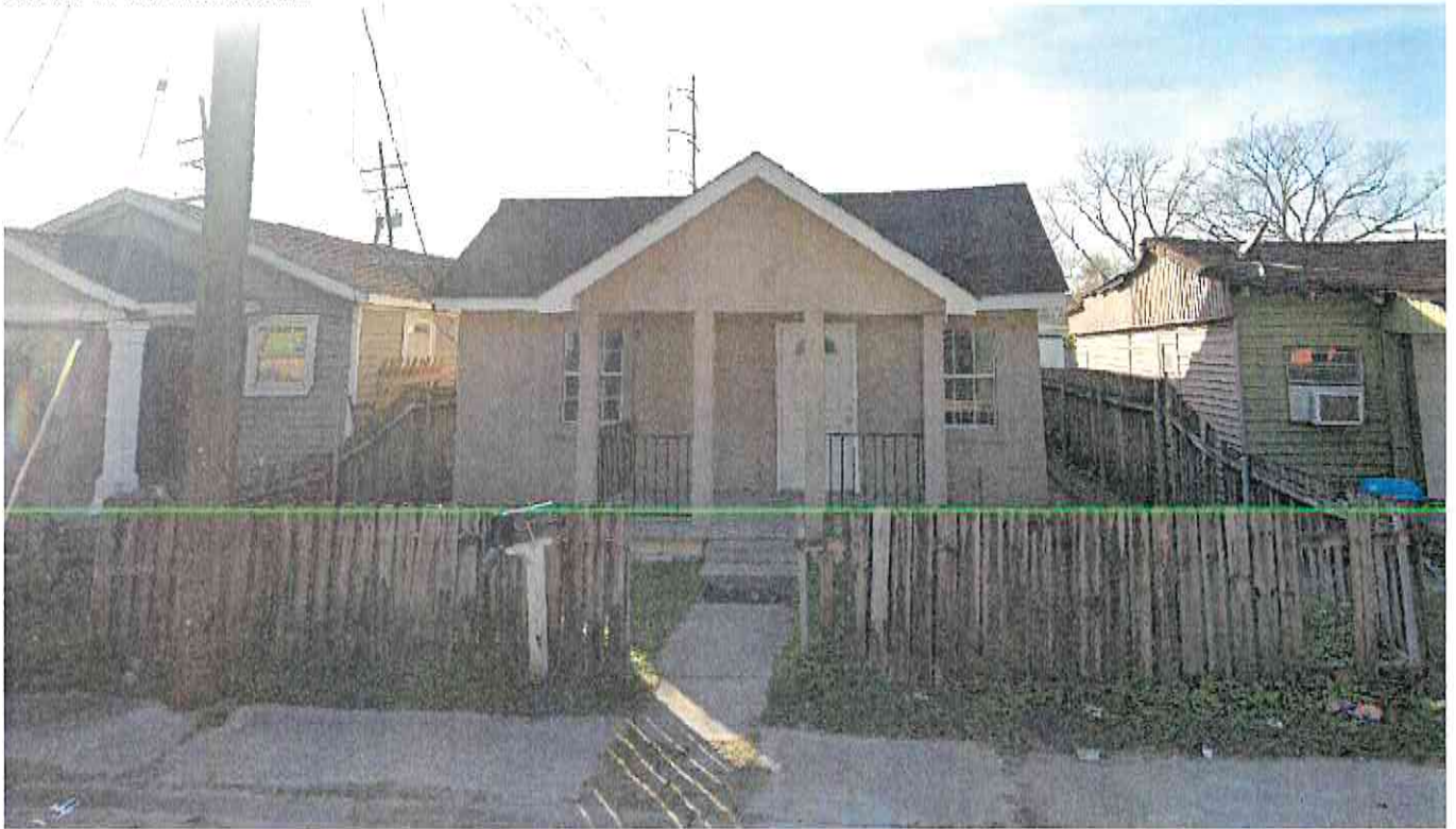
House to be demolished.
