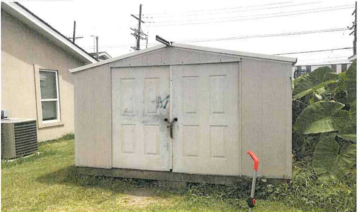
Shed to be demolished.
